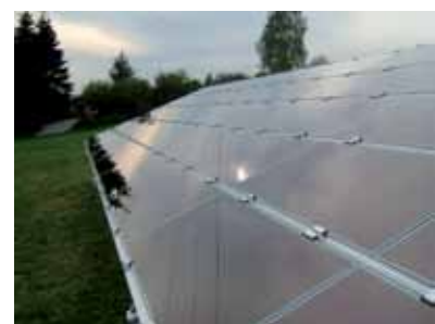
Horizontal mounting of laminated (thin-film) modules
